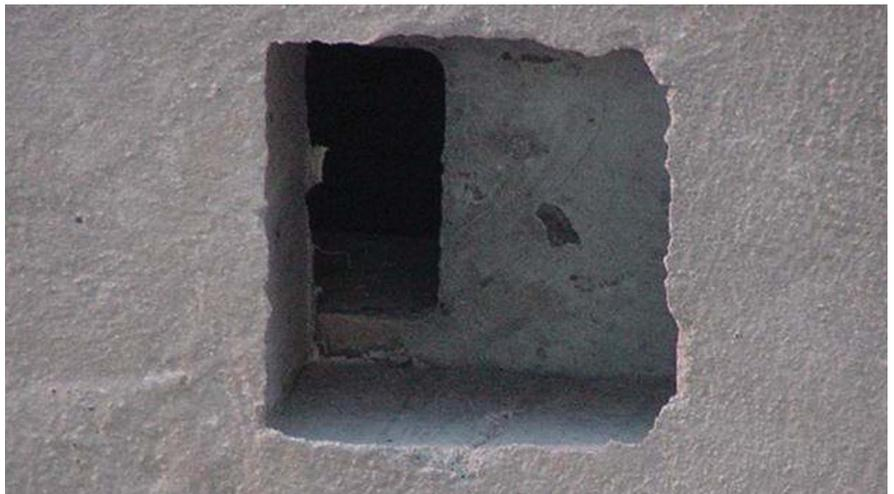
Fig. 10. Misaligned 6 x 6 in. (150 x 150 mm) holes between a precast piece and a cast-in-place wall.
