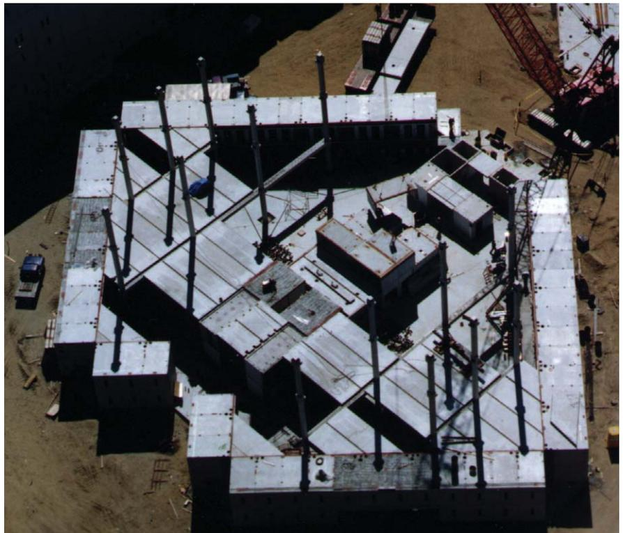
Fig. 9. Prison construction using precast modular cell units.
