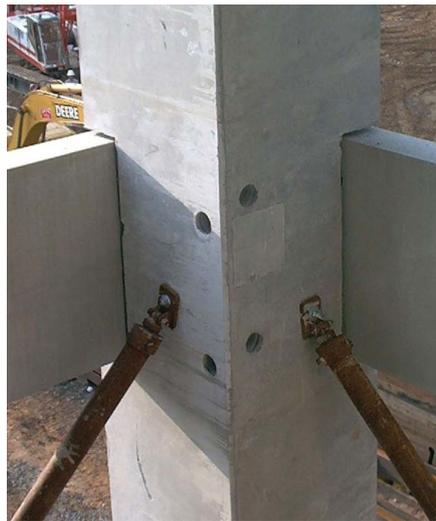
Fig. 8. Spandrel connections to wall and column: as built.
